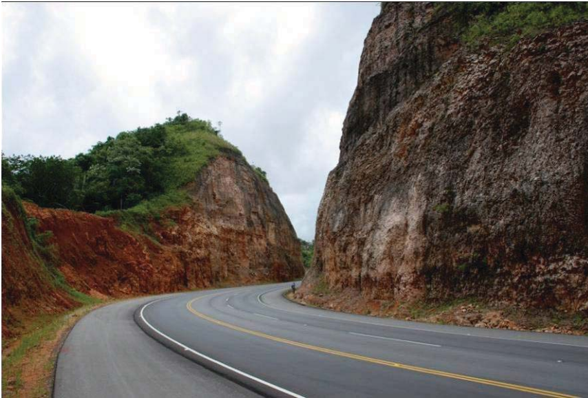
Figure 3: Road cut through Miocene (?) limestone showing the nature of the karst and the formation of pinnacle-like features separated by solution depressions and sinks. Much of the drainage is through subterranean conduits
